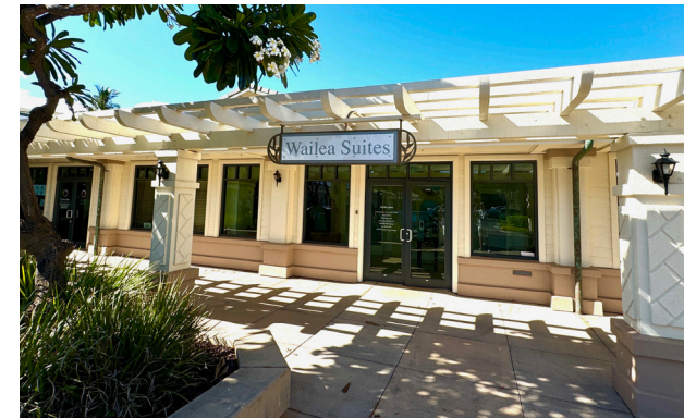
Well-trafficked and established businesses in Building A include 7 Executive Offices at Wailea Suites, Dr. Martin Dermatology, Hansen Realty, and Matteo's Osteria Italian restaurant.
